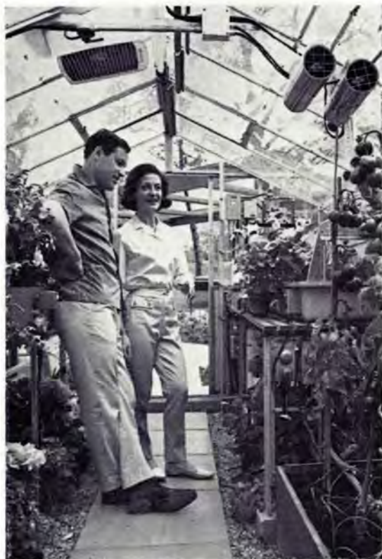
△ The temperature in this greenhouse is maintained automatically at the optimum growing temperature by two aspirated thermostats (top right). One controls an extractor fan (top left) which removes warm air in summer and the other controls the heating.
