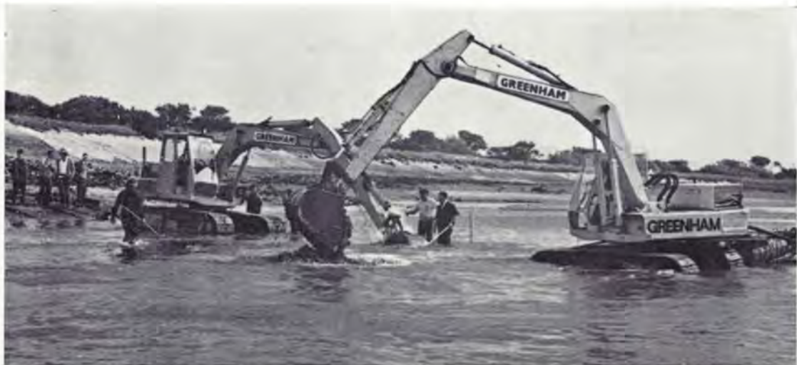
For all the world like a couple of mechanical ducks searching for tit-bits, the two huge excavators are pictured hard at work digging out a trench in the river bed to make the cable's final resting place.
