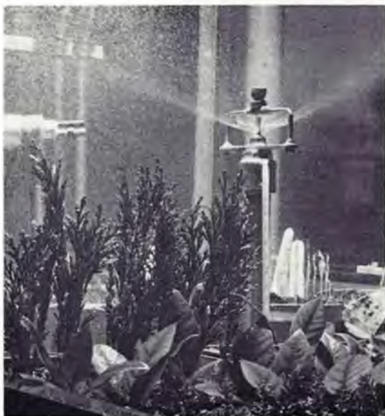
△ The temperature in this greenhouse is maintained automatically at the optimum growing temperature by two aspirated thermostats (top right). One controls an extractor fan (top left) which removes warm air in summer and the other controls the heating.
