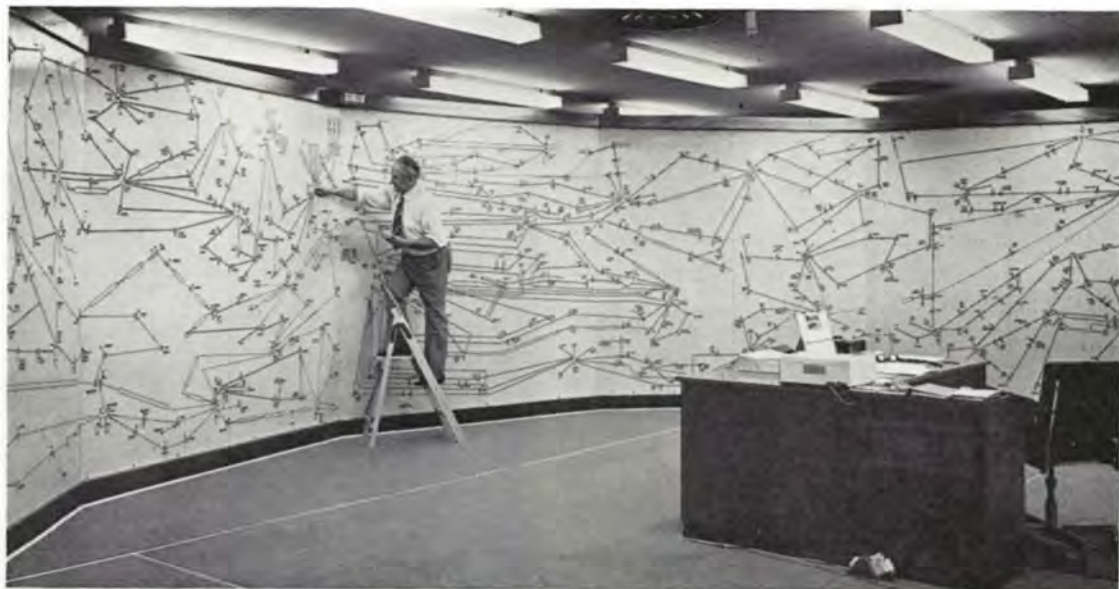
Mr. Cyril Gibson adjusts information symbols on the Reporting Centre's 33kV system diagram to show the current operating condition of the MANWEB 33kV network.
